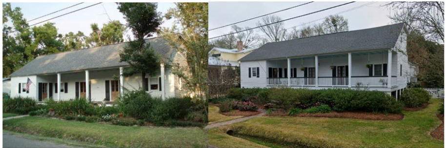
Before elevation (left) and after (right) shows how the retention of historic columns and use of landscaping can minimize the effect of elevation.
