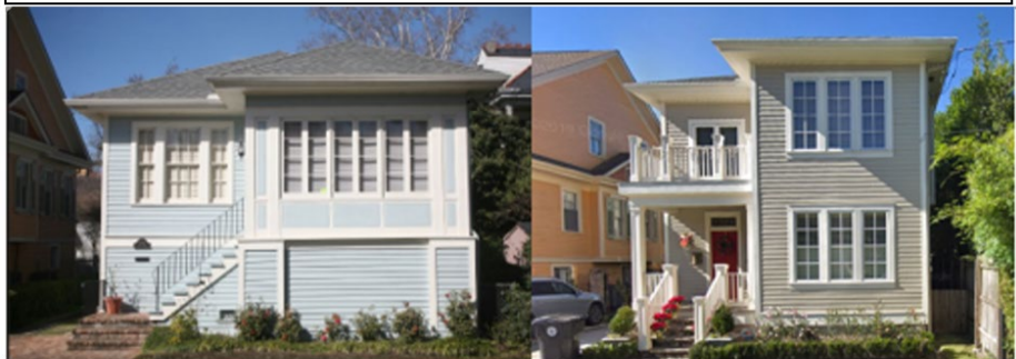
Before elevation (left) and after (right) shows how the introduction of new elements and materials adversely affect a historic property so it is no longer recognizable.
